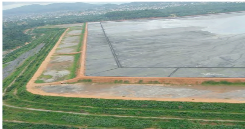
Fig. 1.0: Aerial view of North Embankment of TSF, Sansu AGA, Obuasi
